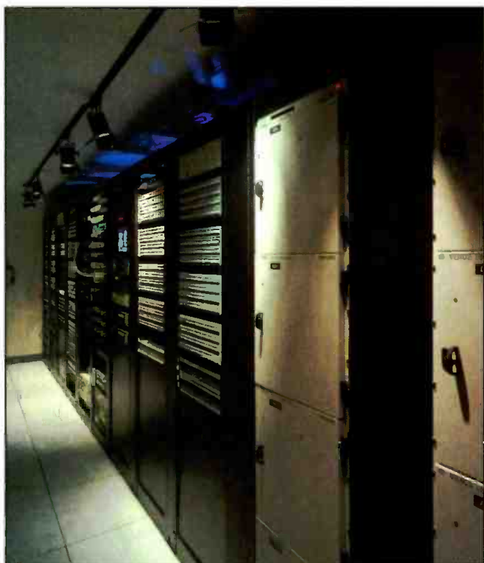
The central equipment room at XETV houses a Venus routing switcher which routes parallel video paths as one to allow easy transition between analog and digital in XETV's operations.
