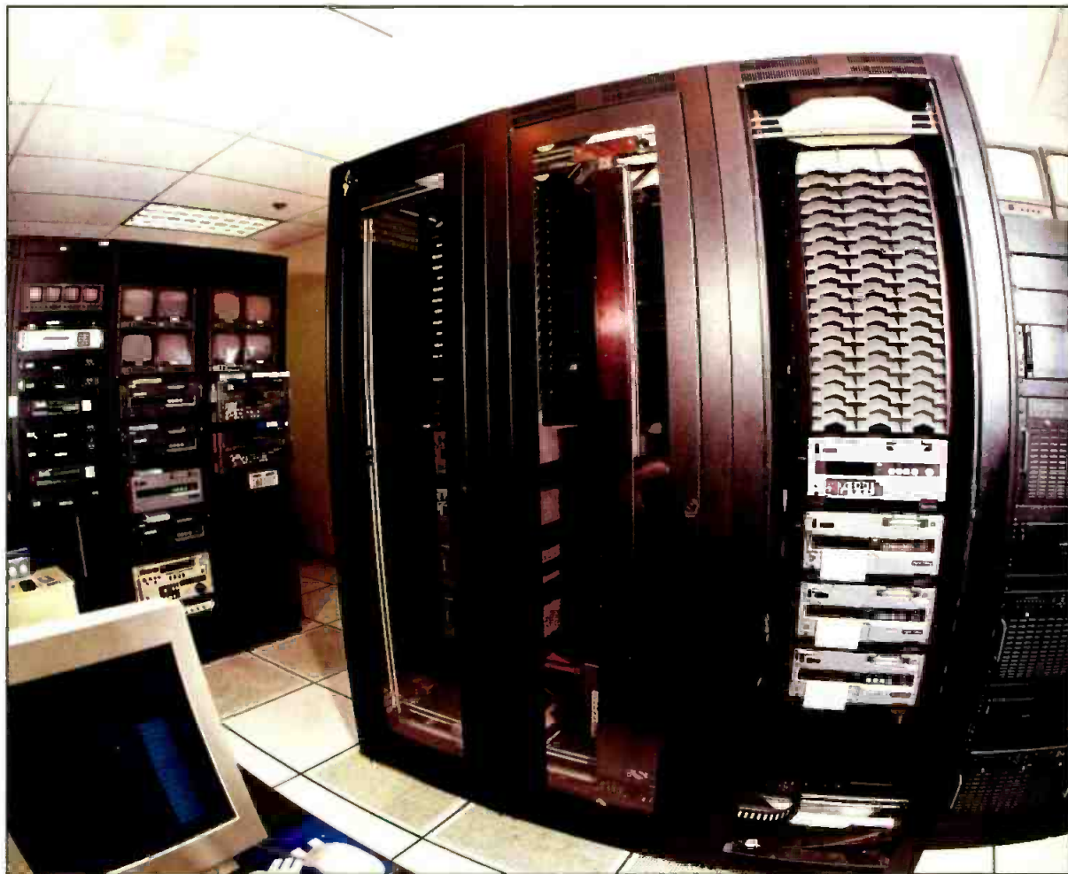
Ackerley's CentralCasting employs a TiltRac V-300 Video Library Manager for its long form and archived program for its regional stations.
